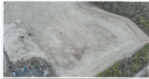
Wa-Ke Hatchee DDMS: Remediated
