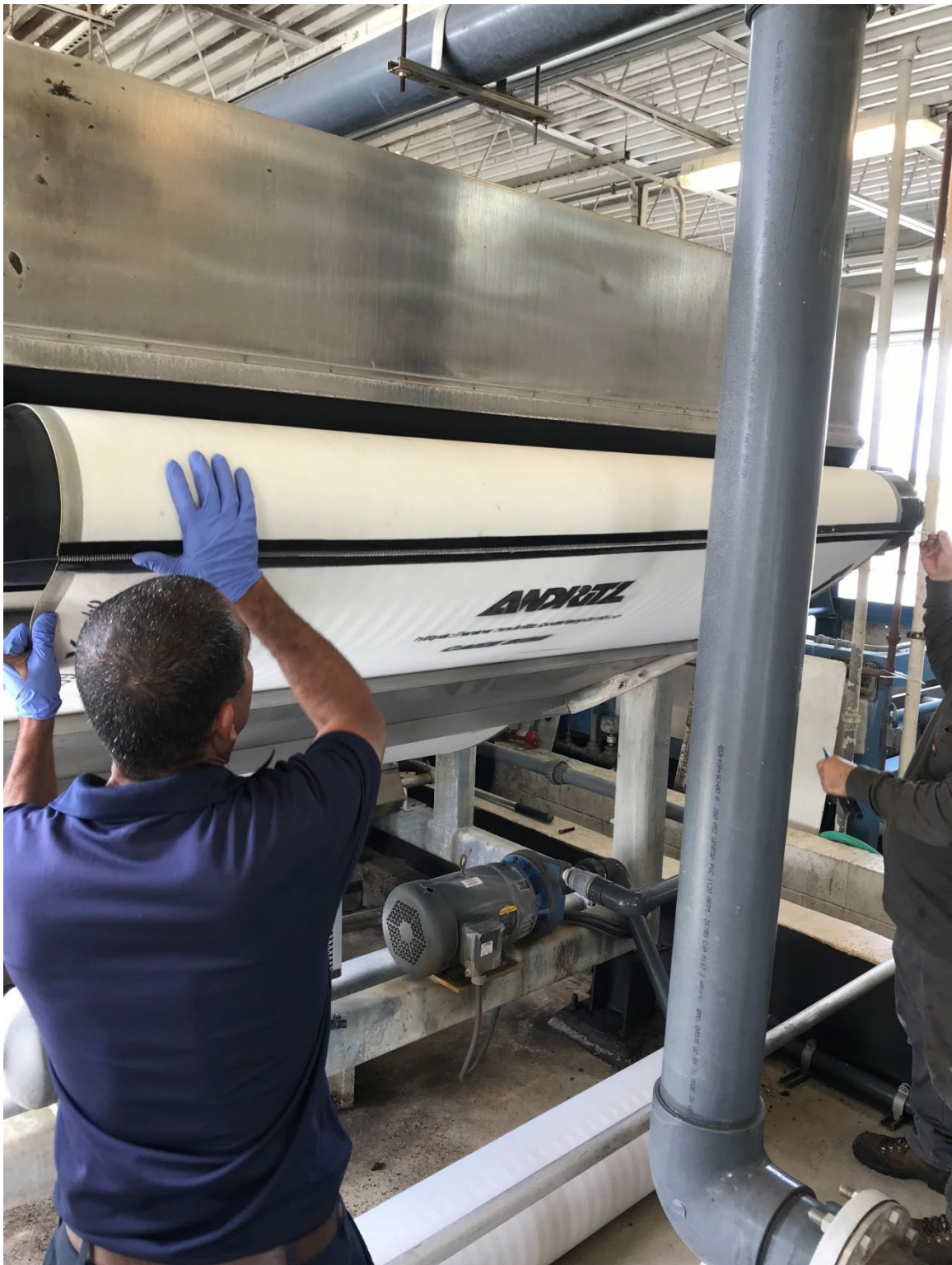
Installing the new lower belt
