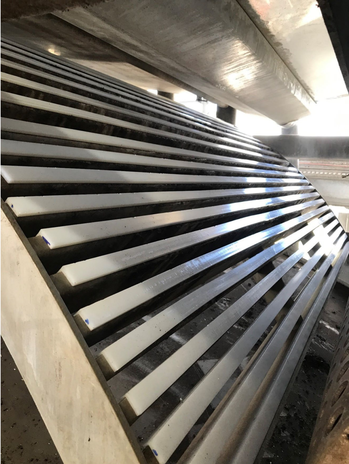
New Teflon wear strips installed
