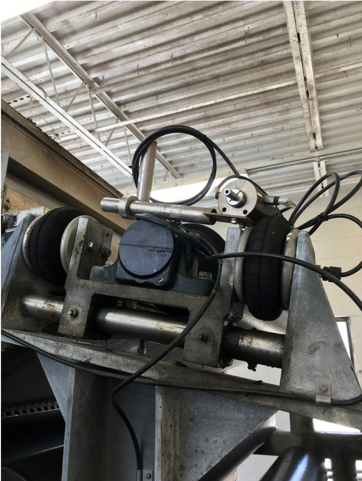
New belt adjusting air bellows installed
