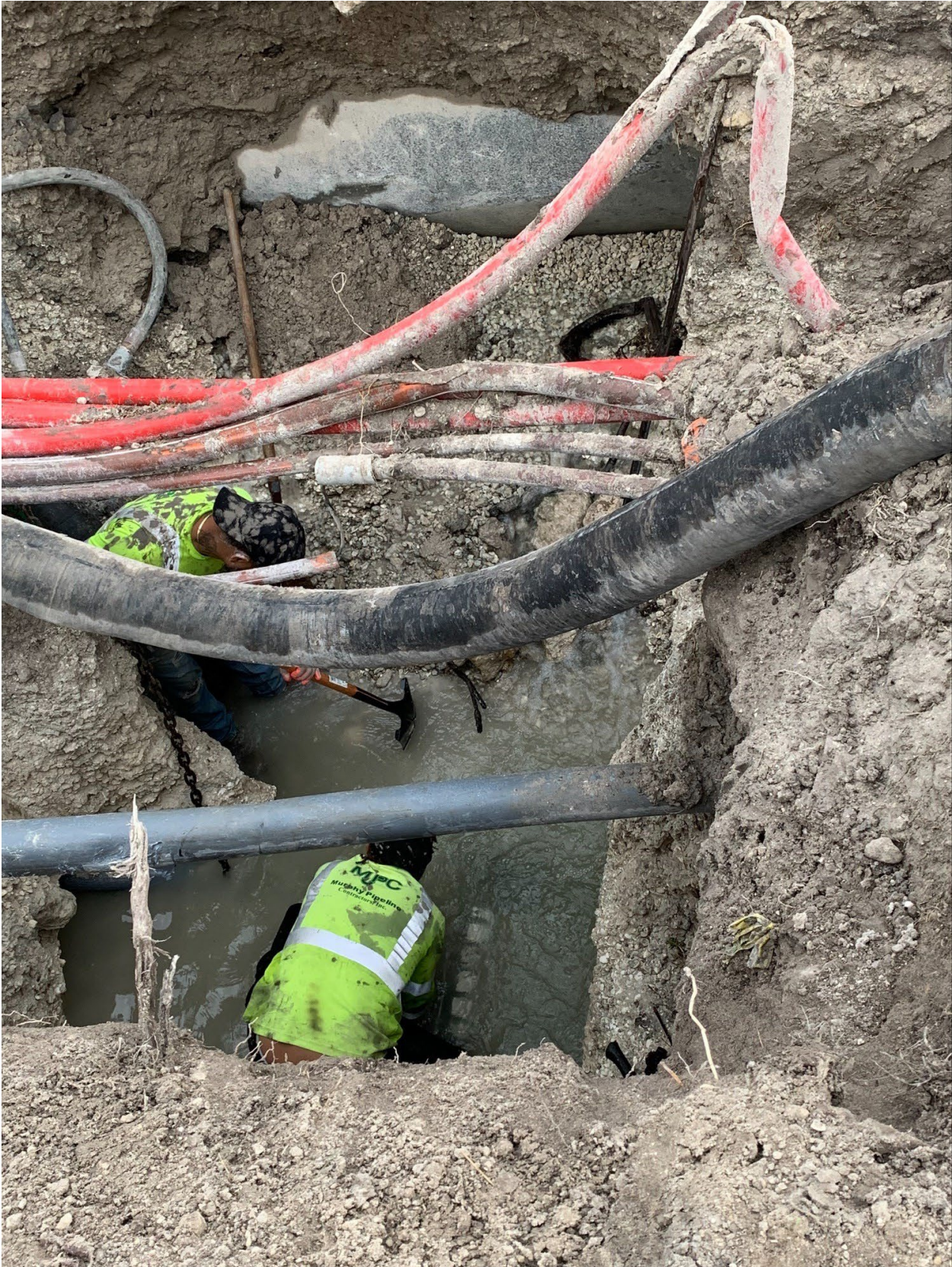
Photos of water main break repair on Atlantic Blvd.
