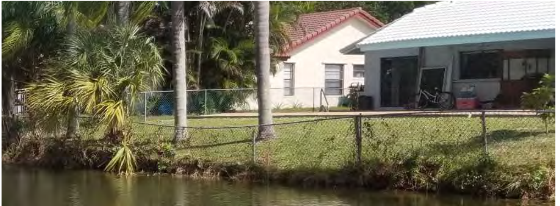
142 NW 110 way-BEFORE REPAIR
