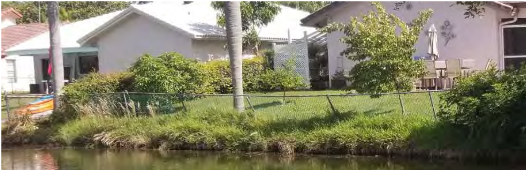
128 NW 110 way-BEFORE REPAIR
